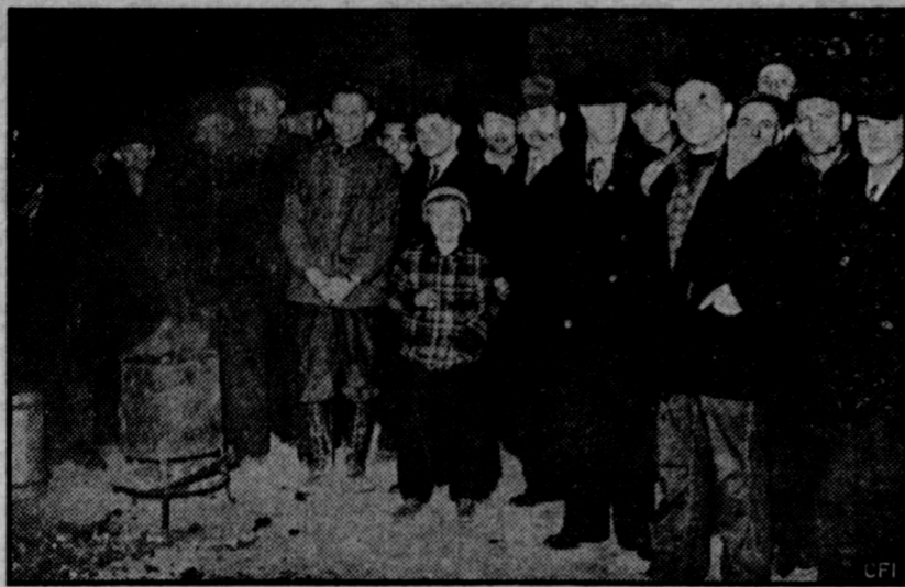
SAGINAW, Mich. April 2.—Striking employees of the Consumers Power Co., took over the operation of an electric generating plant at Zilwaukee, near here, after the company stated that they could not renew its contract with the Utility Workers Organizing Committee, a CIO affiliate. This and other plants are being run without interruption of service and the strikers are awaiting the return of Gov. Murphy for a settlement of their differences. Photo shows a group of strikers picketing the Zilwaukee plant as they are gathered around an improvised campfire to keep warm.
