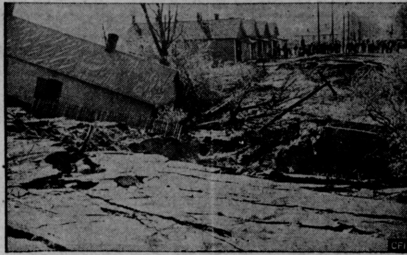
A scene in Owensboro, Kentucky, when a section of Breckenridge Street collapsed following heavy rainfall. A trunk sewer line forty feet below the street surface gave way and the sandy soil began to crumble away endangering several residences in the neighborhood. Many families fled their homes on advice of city officials. The cave in affects an area of about one hundred by two hundred and fifty feet.
