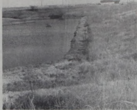
Flood Control dam on Ray and T. Voth farm. Erosion caused by wave action on the front toe of the dam. Shoreline common reed grass was planted on 3 flood control dams this spring to help control wave action erosion at the waterline of earthen dams. Three rows of rhizomes were planted, 40 inches apart, beginning at the waterline and continuing up the slope. Shoreline common reed is a native perennial grass with short, thick rhizomes. The culms are three to eleven feet tall. Stolons usually spread rapidly near the waterline where planting are established. The leaves are 1/2 to 2 inches wide. The seed head is large with many branches and many flowers. The areas planted have to be fenced off because cattle relish the reed grass.
