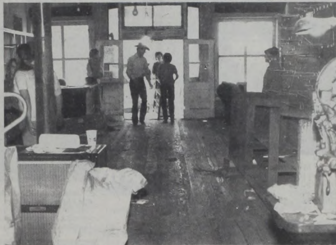
Moving their store from the old to the new location was no problem for Jim and Cindy Gehrig. The job was done for them Sunday between 10 a.m. and 3:30 p.m. by some 60 relatives and friends, most of whom had been at the vacant building Saturday night to celebrate the 65th wedding anniversary of the Matt Mullers, Jim's grandparents. The merchandise was moved a half block down Main Street to the former Pagen Store from the acient Gehrig building, the oldest store in town. Here are near-empty views of the old building.
