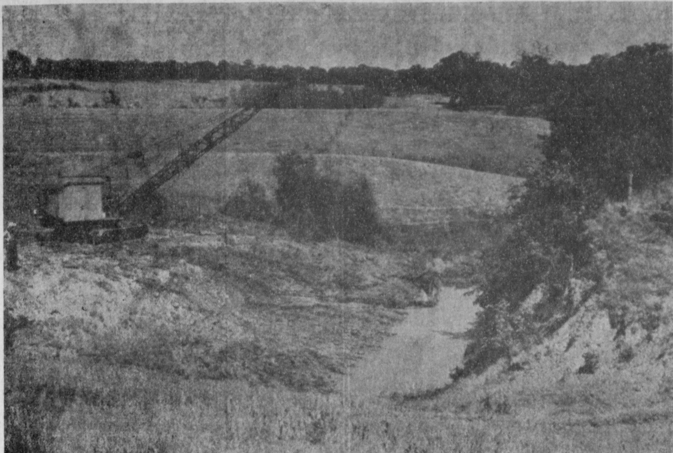
Man-made lakes and dams are in constant need of maintenance to be sure they function according to the design. The back side of this dam eroded before a cover of grass was established. The silt covered the outlet pipe and willows, cattails, and watergrasses added to the problem. Yosten Sand and Gravel Co. of Muenster was employed by the Clear Creek Watershed Authority to do this maintenance job. County commissioners in Cooke and Montague Counties and the Upper Elm Red Soil and Water Conservation District are also sponsors and engage in maintenance work on the dams.
