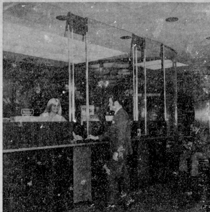
To reduce the chances for robberies, many banks are enclosing the tellers' compartments with sheets of clear Plexiglas acrylic plastic. The acrylic shields deter would-be holdup men without interfering with the normal flow of business.
