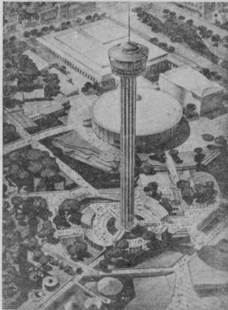
Construction will start in January on the 622-foot Tower of the Americas, the dominant structure planned for HemisFair 1968 in San Antonio. The tower will be built with $5.5 million in general obligation bonds approved overwhelmingly by voters in the HemisFair city. Completion is scheduled for March 1, 1968, five weeks before the April 6 opening of the first major international exposition ever held in the southern half of the United States.
