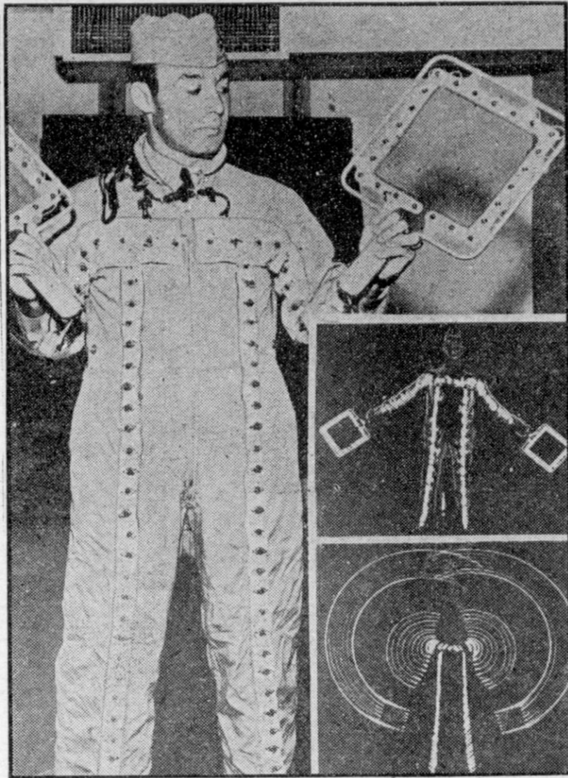
"FLASHY" OUTFIT—Lit up like a Christmas tree, Lt. T. S. Lockard, landing signal officer aboard the USS Midway, models his new suit with tiny light bulbs strung up and down and across his body and signal paddles. Insets at lower right show how he looks to pilots returning to the carrier at night.
