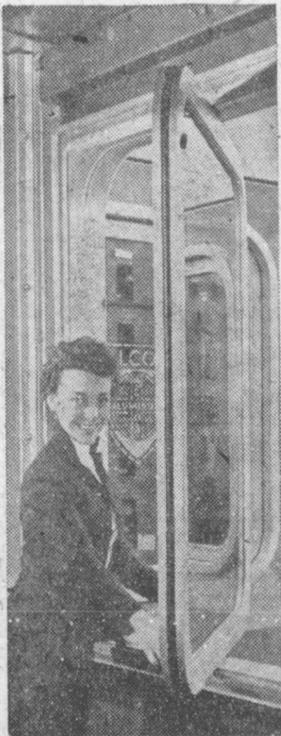
**WASHING WINDOWS** of the ultra-modern Alcoa Building in Pittsburgh, Pa., has been simplified by science. Washing the windows at Alcoa means deflating the butyl tube, swinging the window inside the building for cleaning, then swinging it back into position. The tube, designed by the General Tire & Rubber Company, holds the window in place. No longer need the window-washer dangle precariously from the 42-floor window casing. His is now an inside job.
