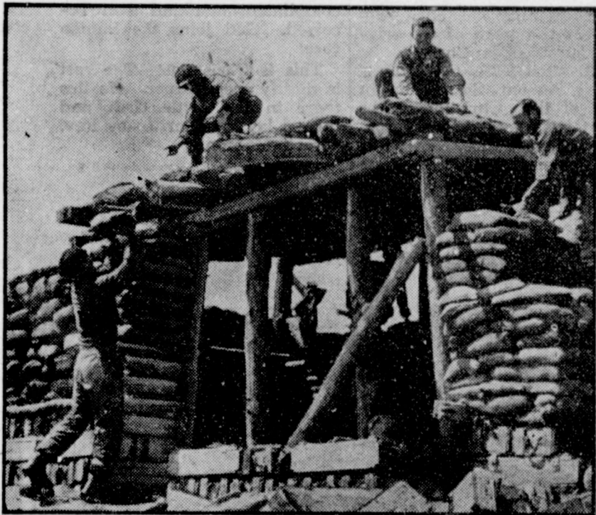
WINNERS OVER WEATHER—Restacking sandbags and rebuilding their bunker near Korean War frontlines, these G.I.'s are busy making the old place more homelike after heavy rains washed out foundations and caved in walls leaving them shelterless.
