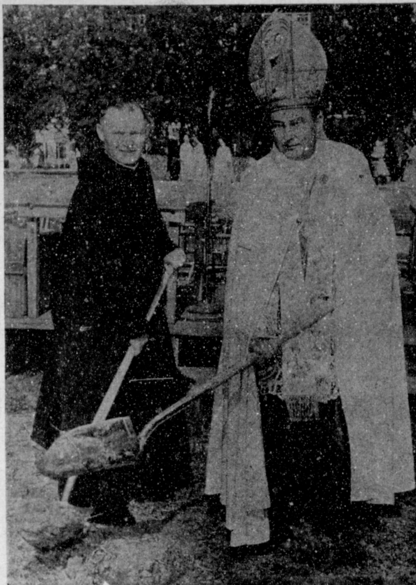
GROUND BROKEN FOR NEW MUESTER CHURCH. The Most Rev. Augustine Danglmayr and Rev. Louis Deuster move a couple of extra shovels full of dirt for Photographer Kent Bellah after the official ground breaking ceremony on Wednesday, May 30, 1952. The new Sacred Heart Church, costing about a half million dollars, will have a seating capacity of 800.
