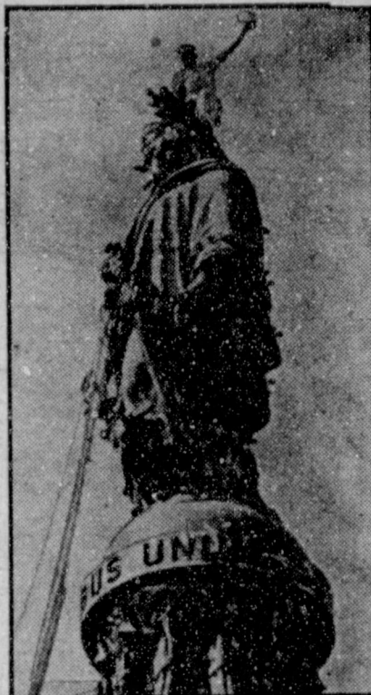
A CAPITOL JOB —From his perch atop the headress of the Statue of Freedom, which tops the dome of the U. S. Capitol Building in Washington, a workman waves to the camera-man who snapped this picture with a telescopic lens. The acrobatic workman was replacing a platinum-tipped lightning rod on the 287-foot-high building.
