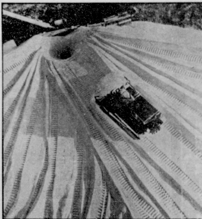
UP THE HILL TO YOUR TABLE—Cutting a swath along the rise a caterpillar tractor pushes salt to the loading pit in Baumberg, Calif. The salt pile is the result of sea water's being pumped into a diked area and evaporated.
