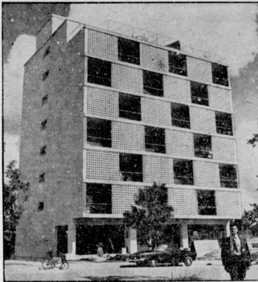
THE BEEHIVE LOOK —With a boom in oil and iron providing big budgets for new homes, apartments and office buildings, Venezuela is witnessing new trends in architecture. The first unit of a development in Caracas displays a beehive brick design which creates a natural air flow and gives protection from the sun. Each studio apartment runs the full width of the building.
