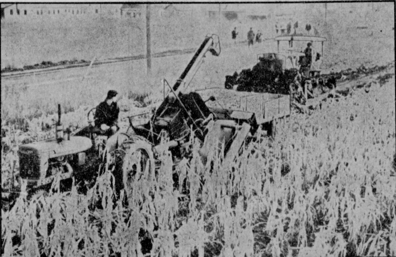
HURRY-UP HARVEST—Farmer Herman Dorris of Flint, Mich., has learned what it's like, at least in one case, when agriculture and industry get together. Informed just 24 hours in advance that construction of a million-square-foot aviation engine plant was to begin on the field he had been renting, Dorris hopped on the tractor which pulled his corn-picker and began harvesting his crop. Here, a few feet in back of his corn-picker, a bull-dozer levels ground for the new building.
