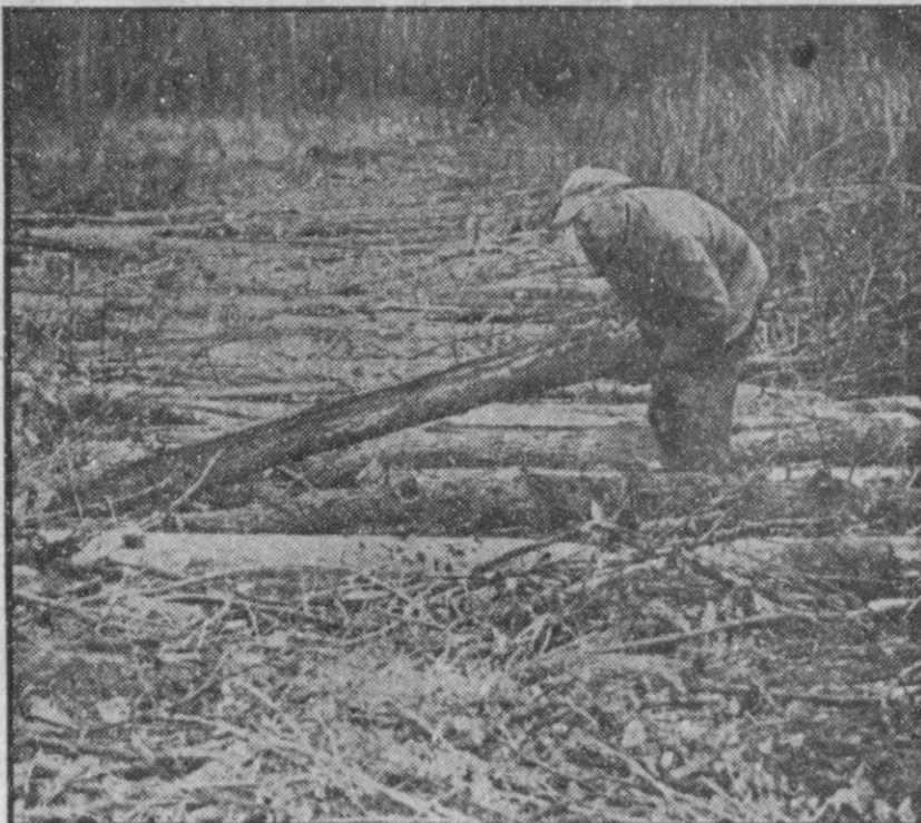
CORDUROY ROAD —Ray Parker of Wayland, Mich., is proving that corduroy roads still have their place in the rural scene by building one. Equipped with modern tools, Parker is constructing an 1800-foot road through a swamp to serve his resort on Gun Lake. He cuts logs, knits them together over a base of small brush, adds a top layer of poles and covers it all with gravel.
