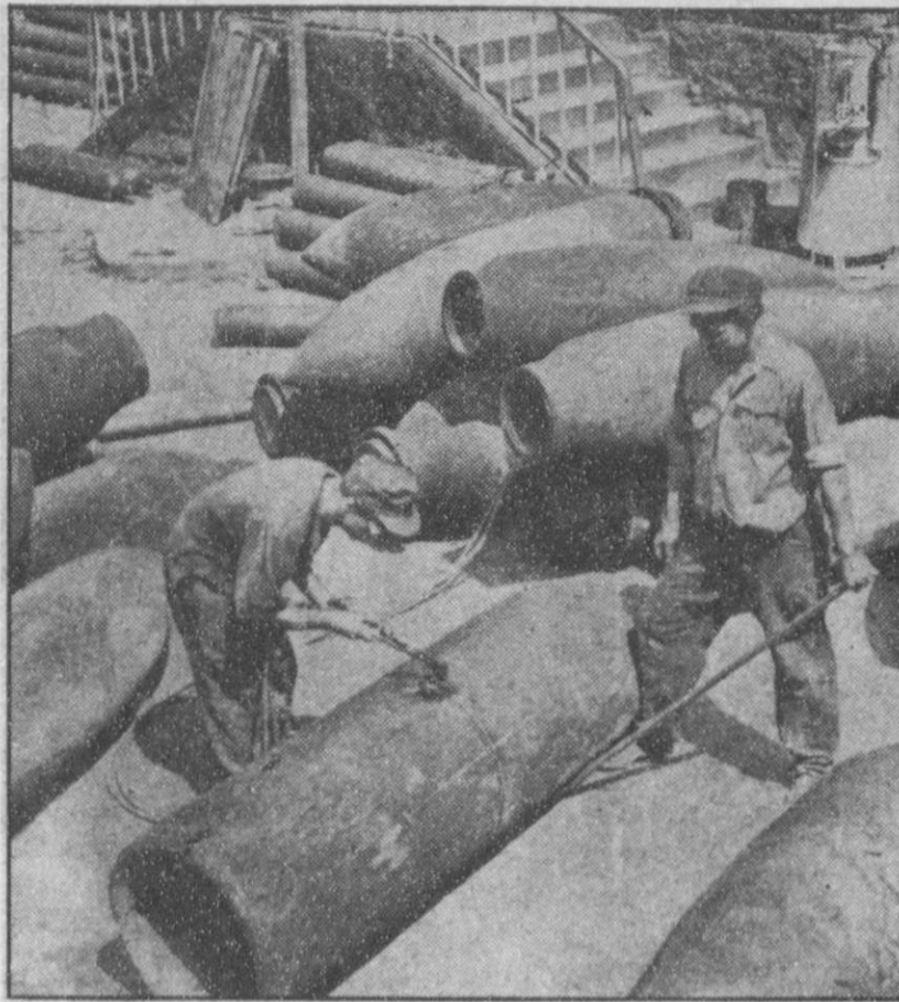
LEFT OVER FROM THE BLITZ —Workmen in Berlin use an acetylene torch to carve up a two-and-a-half-ton blockbuster for scrap. Originally destined for England via the Luftwaffe, the bombs are among hundreds of tons of scrap iron and steel being shipped daily to England by a more peaceful water route.
