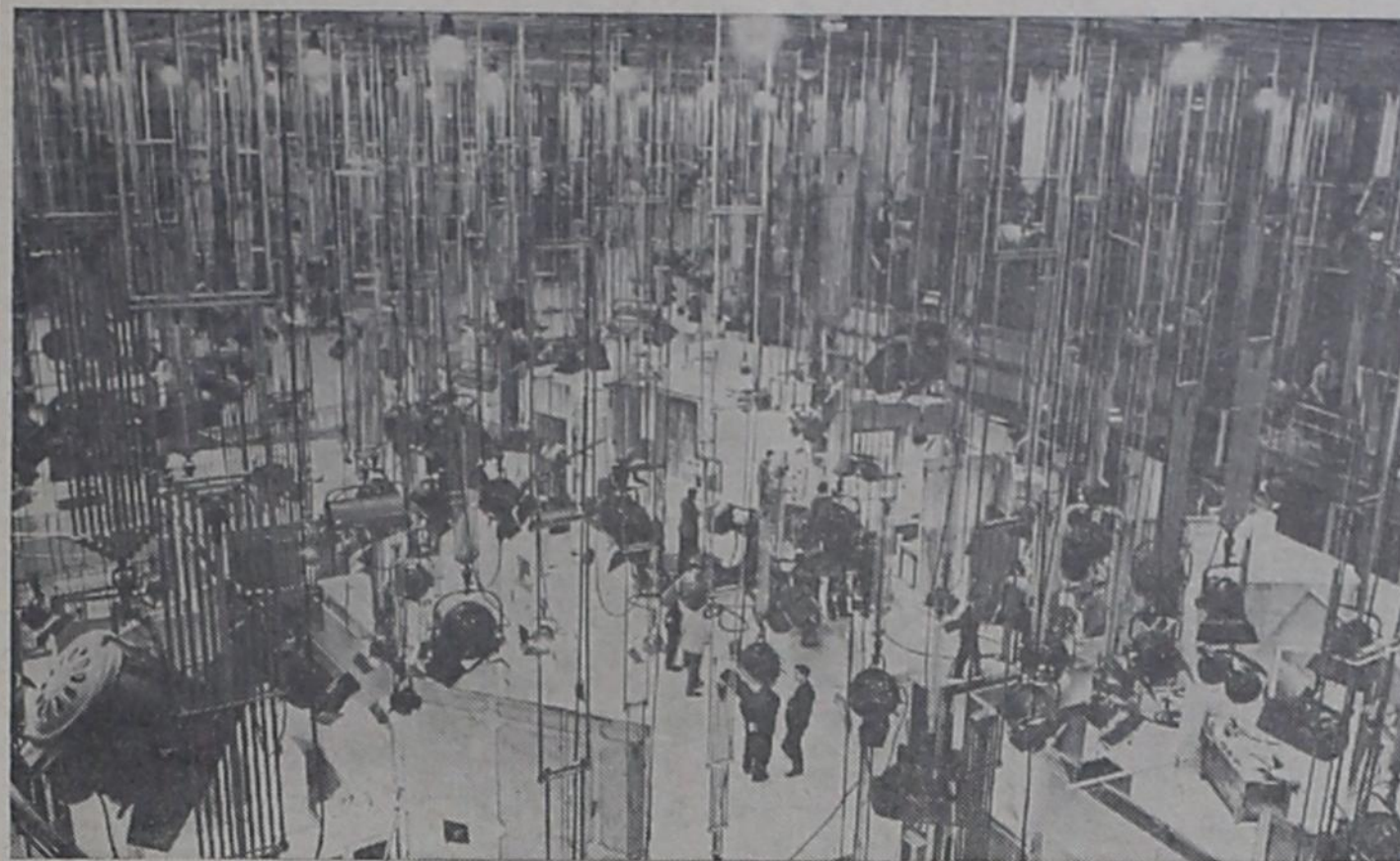
ELECTRONIC CURTAIN —A new television studio at Elstree, England, seems hidden by a curtain of metal rods. The curtainlike complex is for camera lights.
