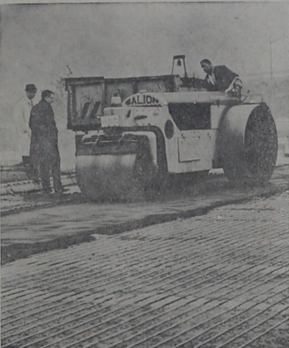
HOT ROAD —A roller helps to cover electrical cables near Newark, N.J., for an "under actual conditions" test of an effective way to heat highways to keep them free of snow.
