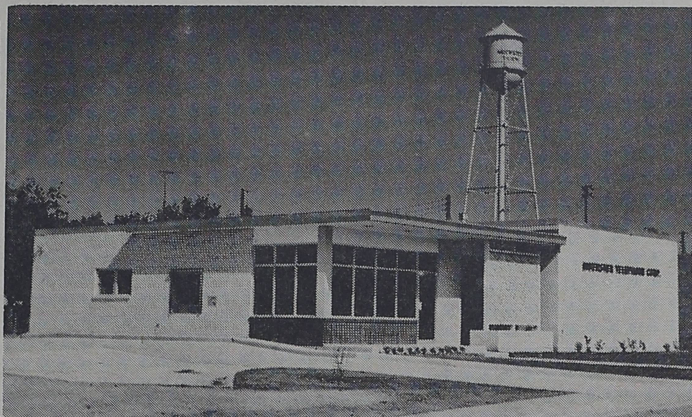
MUENSTER TELEPHONE CORPORATION'S new building has been used as an office since this week Monday and will go into use as an exchange at 2 o'clock Saturday when the change-over to its new automatic equipment will mark the beginning of dial phone service here.
