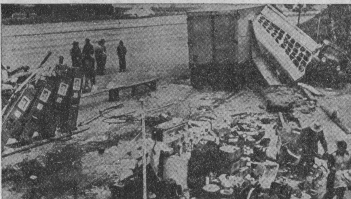
BRISBANE, CALIF.—(Soundphoto)—Tilted gas pumps and mass of debris are all that is left of steel-frame gas station here after it was hurled off its foundation and carried 20 feet when a huge 15-wheel truck-trailer veered off Bayshore highway and smashed through it. John Vincequerra, 24, San Jose Calif., the truck driver, said two automobiles in front of him suddenly stopped directly in his path. He applied airbrakes, but they failed, and he swerved to avoid hitting the cars. The truck plunged across curbing and into gas station, carrying it with it before coming to rest (rear) against hill.
