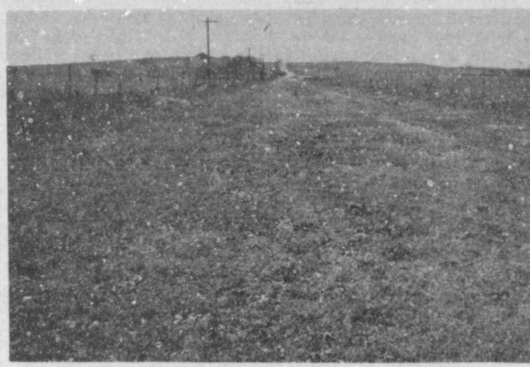
A WATERWAY, BEFORE AND AFTER. Pictures show an old abandoned road (above) that was shaped, and sodded to Bermudagrass for a diversion terrace outlet, on the Alois Trubenbach place. The diversion terrace, which was built this spring, keeps runoff water from 100 acres of pasture land on cutting across good bottomland field on the right of photo. Many such waterway-terrace combinations are needed in the Muenster area to protect good cultivated land from erosion.
