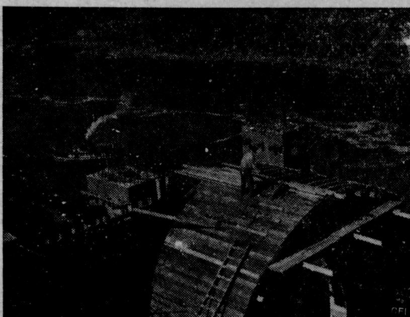
NIAGARA FALLS.—White bridges on International Borders in Europe are being destroyed, first concrete arches of Rainbow Bridge, 200 feet above famous gorge, take form from Canadian and New York shores.
