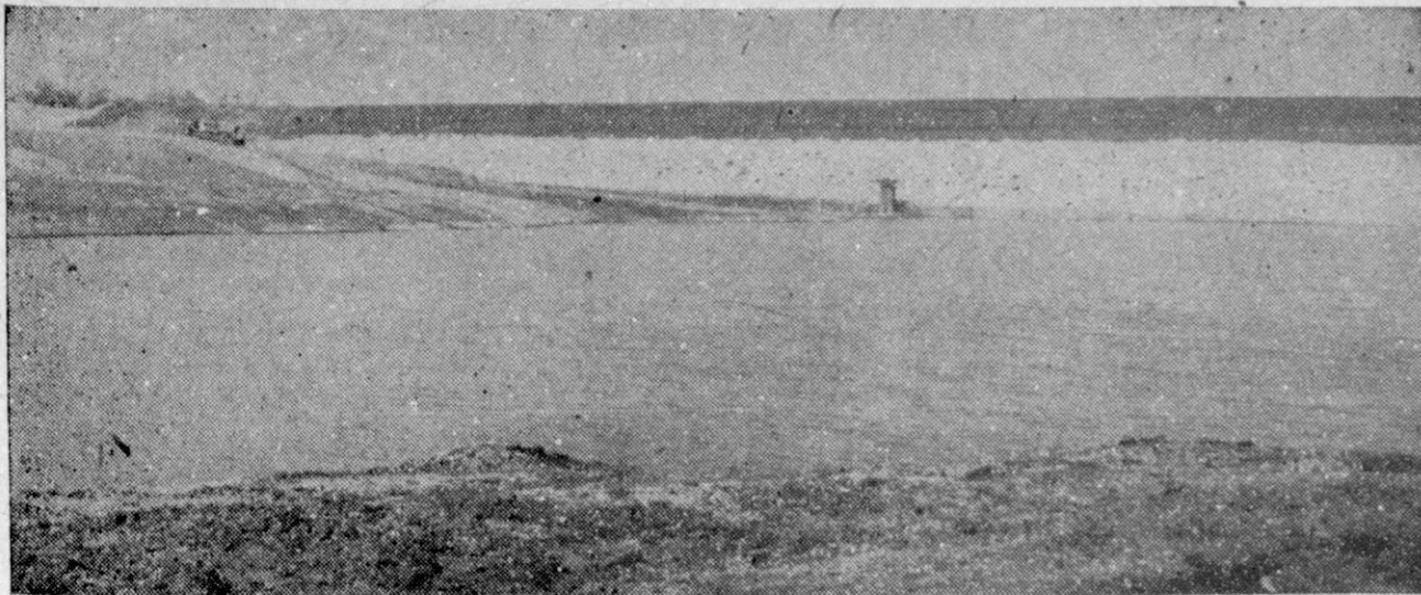
FLOOD PREVENTION RESERVOIR on the Joe Fisher farm. Dam is located on Squirrel creek, a tributary of Upper Dry Elm near the home of Henry Pick. View is looking across the reservoir area toward the rock faced dam. The concrete inlet structure is visible in the center of the dam. Spillway is on the extreme left side of photo. The dam was completed on April 12. Ten days later it was filled to within a few feet of the emergency spillway.
