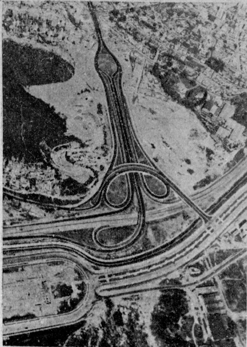
FOLLOW YOUR NOSE —This complex loop-the-loop highway pattern illustrates the modern look along a 550-mile stretch of Venezuela's section of the Pan-American Highway leading into Caracas. Now completely paved, the road has reduced driving time from Caracas to the Colombian border to 15 hours. Previously, it was a two-day trip. Speeds of up to 80 miles an hour are permitted on many stretches. It's part of Venezuela's booming public works program.
