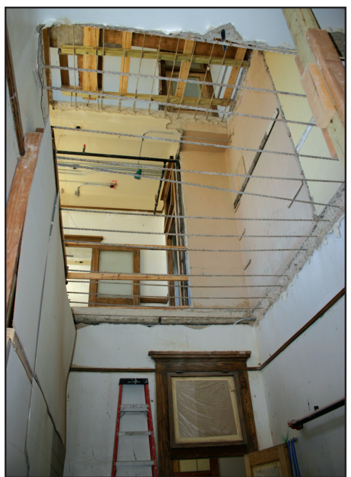
Work continues to progress in the Cooke County Courthouse. Shown above is scaffolding reaching from the basement to the ceiling where the beautiful stained glass was removed for cleaning. Below, at right - floors were removed to put in fire escape stairs to replace the outside slides for escape; at left - the second floor ceiling was removed to restore this portion to its original high ceiling design. Janie Hartman photos
