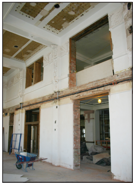
Work continues to progress in the Cooke County Courthouse. Shown above is scaffolding reaching from the basement to the ceiling where the beautiful stained glass was removed for cleaning. Below, at right - floors were removed to put in fire escape stairs to replace the outside slides for escape; at left - the second floor ceiling was removed to restore this portion to its original high ceiling design. Janie Hartman photos
