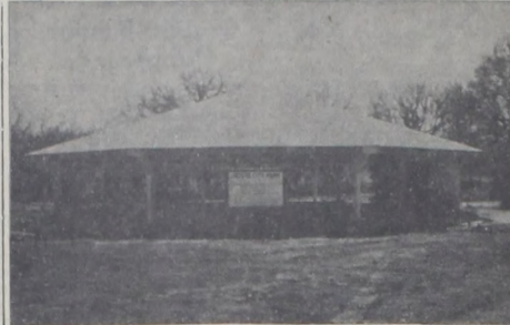
This pavilion in the city park is the inspiration behind the bull ride sponsored Thursday, Friday and Saturday nights in the Twin Pines inside arena by Muenster Jaycees. Proceeds from the show will be applied to the Jaycees debt on the project. Thursday is kids night at the bull ride. Youngsters under 12 will be admitted free if accompanied by a parent.
