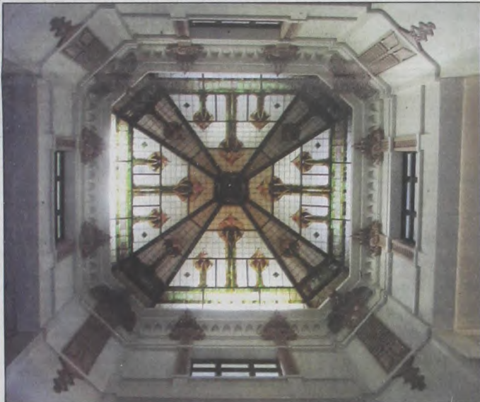
The stained glass dome of the Cooke County Courthouse lights up the center rotunda of the empty building. With all officials, files, and newer furniture moved out to temporary locations, the Courthouse is now ready for its interior restoration to begin. See page 3 for more pictures of the vacant historical structure. Janie Hartman photo
