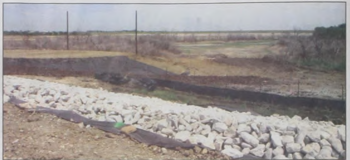
Layers of rip-rap rock have been hauled on and around the Muenster Lake parking lot area as work continues at the west side entrance. The boat ramp will descend off the lot from between the two high-line poles. The parking area will also allow easy access to the walking trails and other future improvements. Janie Hartman photo
