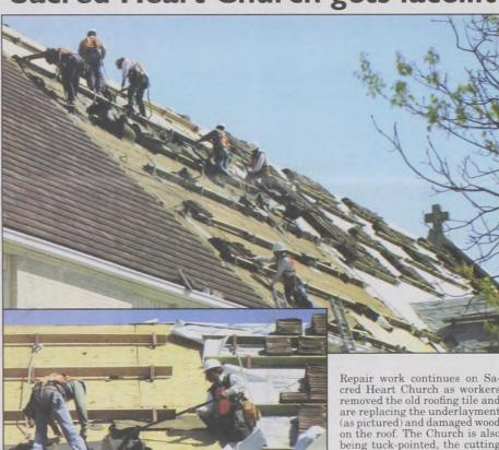
Repair work continues on Sacred Heart Church as workers removed the old roofing tile and are replacing the underlayment (as pictured) and damaged wood on the roof. The Church is also being tuck-pointed, the cutting out of old mortar and replacing it with new ut of our mo-with new. Janie Hartman photos
