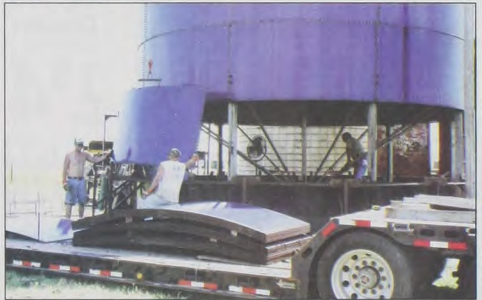
A change in the skyline north of Muenster took place Tuesday afternoon as the 80' Harvester erected by Arnie Knabe on his dairy farm came down. The tall landmark stood for 35 years and could be seen for many miles. A crew dismantled the tank from the bottom. It was assembled in this same manner years ago. The storage tank was no longer used for feed and was sold by Aileen Knabe. At left, nuts are loosened and bolts taken out. Above - the curved panels are taken down one at a time. Below - as each level was finished, the Harvester pieces were loaded on a trailer for transport to a new location where the tank will be reassembled. Janie Hartman photo
