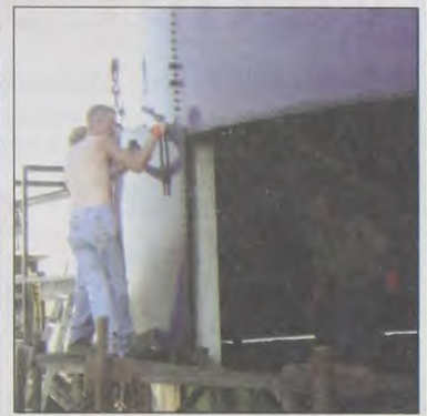
A change in the skyline north of Muenster took place Tuesday afternoon as the 80' Harvester erected by Arnie Knabe on his dairy farm came down. The tall landmark stood for 35 years and could be seen for many miles. A crew dismantled the tank from the bottom. It was assembled in this same manner years ago. The storage tank was no longer used for feed and was sold by Aileen Knabe. At left, nuts are loosened and bolts taken out. Above - the curved panels are taken down one at a time. Below - as each level was finished, the Harvester pieces were loaded on a trailer for transport to a new location where the tank will be reassembled. Janie Hartman photo
