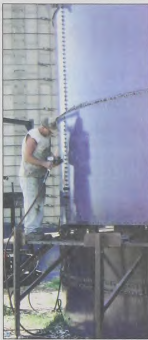
A change in the skyline north of Muenster took place Tuesday afternoon as the 80' Harvester erected by Arnie Knabe on his dairy farm came down. The tall landmark stood for 35 years and could be seen for many miles. A crew dismantled the tank from the bottom. It was assembled in this same manner years ago. The storage tank was no longer used for feed and was sold by Aileen Knabe. At left, nuts are loosened and bolts taken out. Above - the curved panels are taken down one at a time. Below - as each level was finished, the Harvester pieces were loaded on a trailer for transport to a new location where the tank will be reassembled. Janie Hartman photo
