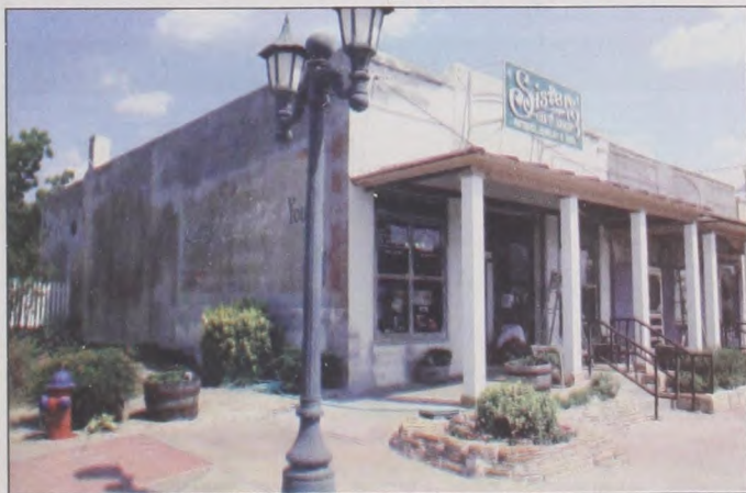
Jan Walterscheid, owner of Sisters Gift Shop, continues the repairs and remodeling of the "Old Gehrig Building" on Main Street. The building was built in 1911 by John Gehrig and was constructed without the use of cement, only lime and sand. It housed Gehrig's Store until 1980. Sisters is open for business during the remodeling. Janie Hartman photo
