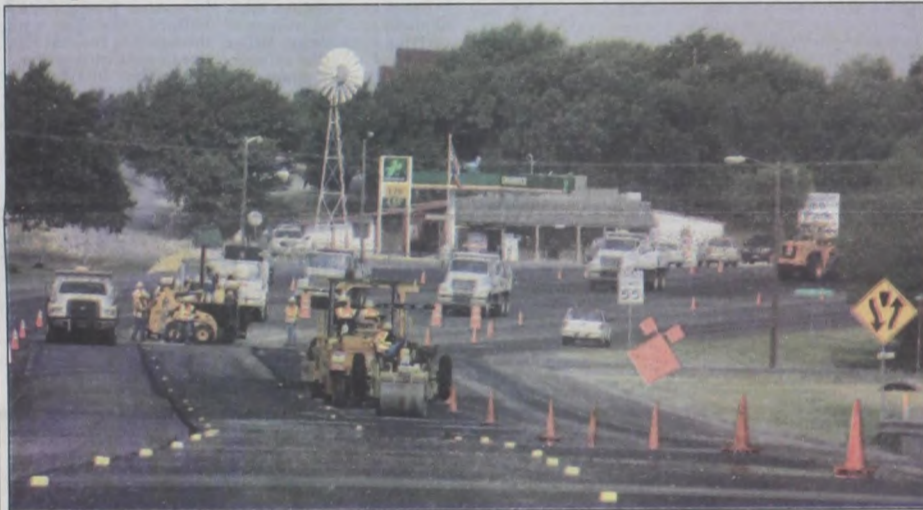
TxDOT finally got around to the resurfacing of Hwy. 82 through town this week after two other paving attempts failed in the last year. Muenster residents have had to deal with humps, bumps, holes, and dust before this overlay of hot mix asphalt was put down, making a smooth driving surface. Janie Hartman photo
