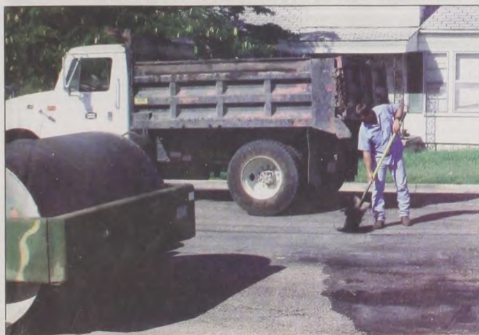
Machinery and manpower teamed up earlier this week to patch City streets in preparation for paving. At left, City worker Rick Hennigan takes care of the smaller problems, while David Dittfurth (above) patches a larger area on South Walnut Street. Janie Hartman photos
