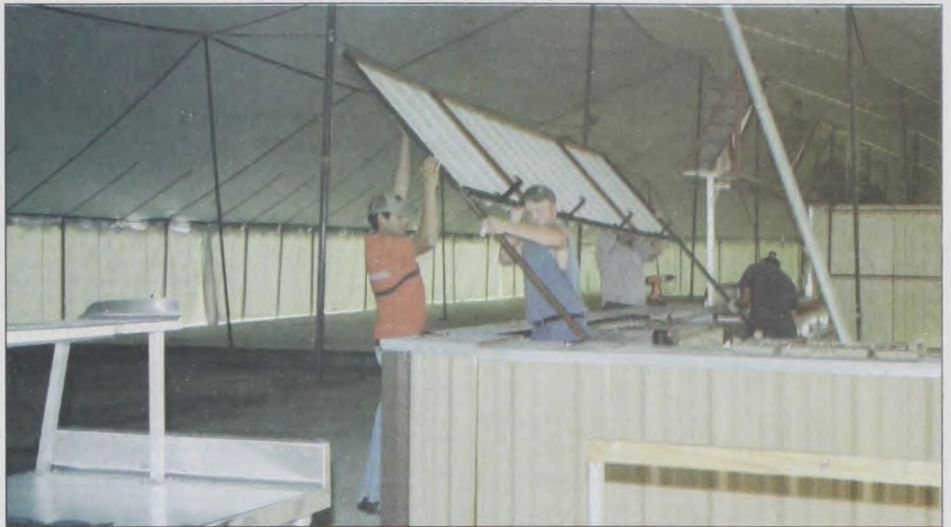
A crew works on assembling a booth for Walterscheid Meat Company inside the big tent earlier this week when the tent was almost empty. Construction of booths inside the tent continued in preparation for this weekend's Annual Germanfest. See special Germanfest insert inside. Janie Hartman photo
