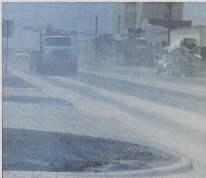
Record breaking temperatures Monday caused oil to ooze out of the pavement on Highway 82 through town. TXDot spread crushed gravel, which kicks up dust, making that section of town look like the dust bowl. Last summer the routine seal coating maintenance job to the highway turned into a bumpy surface until the end of October when the seal coat was removed and a temporary chip and tar surface was put down. That surface is once again getting very bumpy as shown below. Janie Hartman photos
