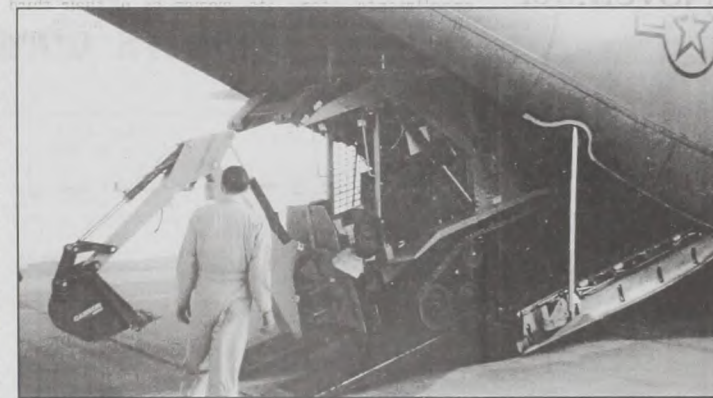
Loading a remote controlled unmanned track hoe used for repairing runways.
