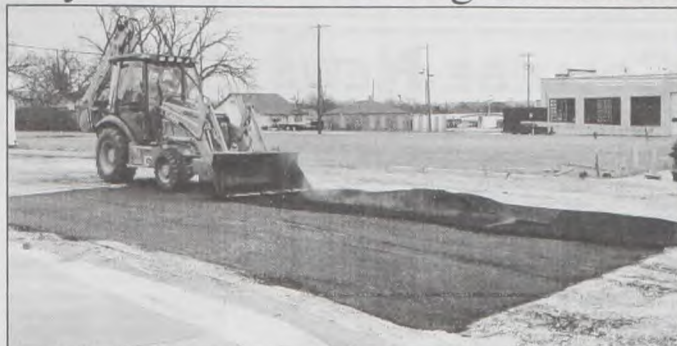
Muenster City employees have been busy patching streets around town in a constant battle against pot holes and damaged pavement. The city's two year plan developed for street improvements has begun with the patch work. Janie Hartman photo
