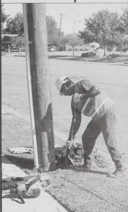
Alfredo Rodriguez performs a highline pole inspection on Main St. The Osmose Co. of Buffalo, NY is conducting the inspection of electric highline poles in Muenster this week. The poles are being checked top to bottom for decay, treated, and then sheathed in a protective wrap below ground level to extend the life of the pole. Phil Keil photo
