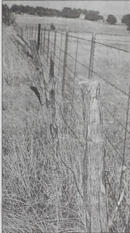
An old bois d'arc farm fence held its ground for many years, but recently lost its strength and was replaced by a newer steel T-post fence. Janie Hartman photo
