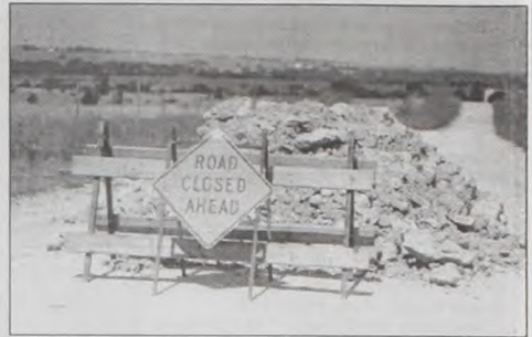
Precinct #4 road crews piled rocks across CR 424 as a second warning to motorists not to travel any further. There was danger ahead caused by a washed out road culvert. Janie Hartman photo
