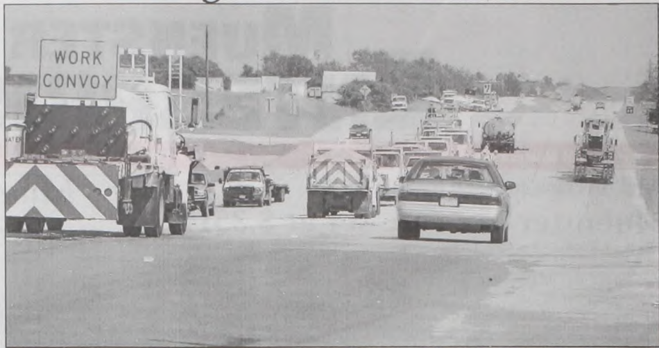
TXDOT continues to work on Hwy. 82 through the center of Muenster. Wednesday's traffic had to work around a line of trucks putting gravel down in the center turning lane.
