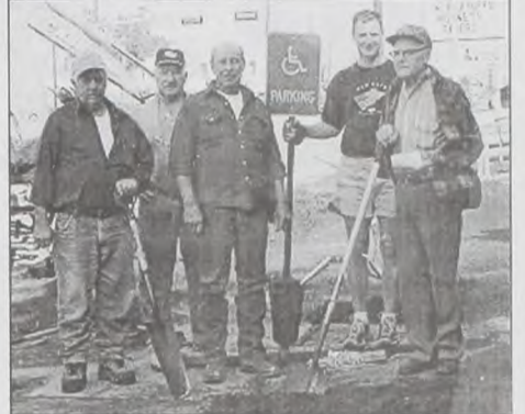
Muenster VFW Post #6205 gets a head start on the Great American Cleanup. G & H Backhoe donated crushed rock, equipment, and manpower to help VFW volunteers landscape and beautify the VFW Post on Main Street in Muenster. Volunteers shown are Bernard Hesse, Leonard Vogel, Herman Grewing, Joe Bright, and Johnny Rohmer.
