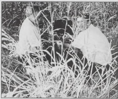
Bob Williams and Jerry Yosten repairing damaged telephone pedestal. Courtesy photo
