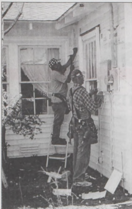
Improvements continue at the Ben and Aggie Seyler Muenster Museum. Ted Hackett and Preston Smith of Hackett Custom Siding are covering the old wood on the house with metal siding. The Muenster Historical Commission is having a fundraiser bake sale this Saturday at Fischer's Meat Market to help cover the cost of the project. Janie Hartman photo
