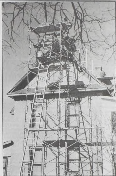
Renovation of the Sacred Heart rectory continues as workers do repair work on the chimneys this week. Removing the stack and rebuilding it to its original status will give the historical building a new fresh look while keeping it in the old style. Janie Hartman photo
