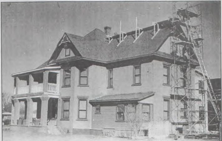
Renovation of the Sacred Heart rectory continues as workers do repair work on the chimneys this week. Removing the stack and rebuilding it to its original status will give the historical building a new fresh look while keeping it in the old style. Janie Hartman photo
