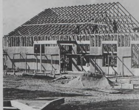
Swift work on the new post office
