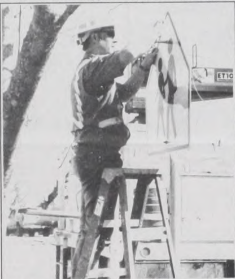
Lee Adams, Texas Highway Department, installs new school crossing signs on Main Street earlier this week. The high intensity fluorescent yellow school signs replaced the old "orange" signs. The new color should draw awareness to drivers that they are approaching the school zone. Photo by Janie Hartman
