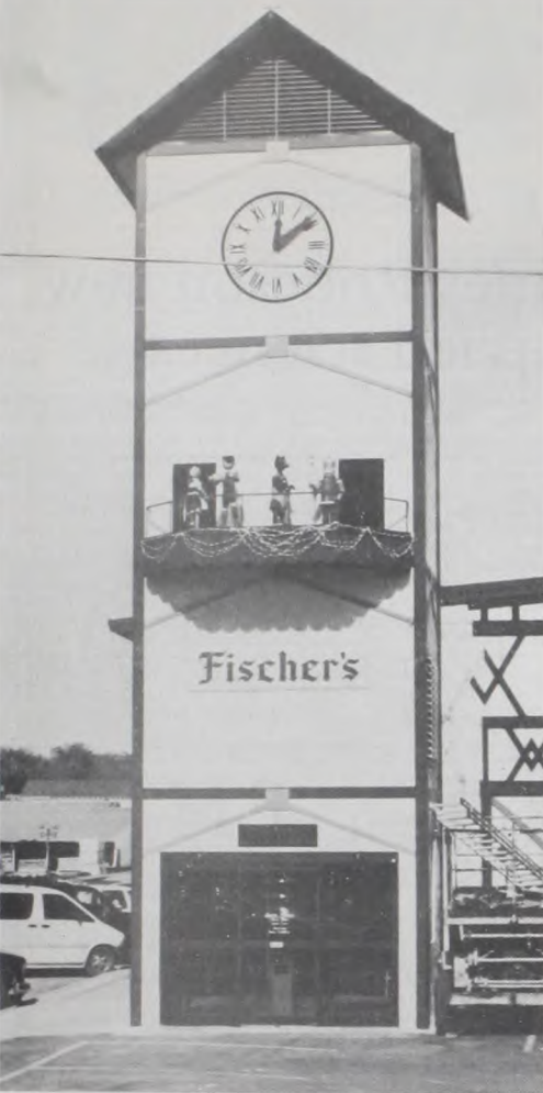
The south entrance to Fischer's Meat Market is dominated by the impressive clock tower that points upward for 40 feet to present the Glockenspiel and its seven traditional characters.
