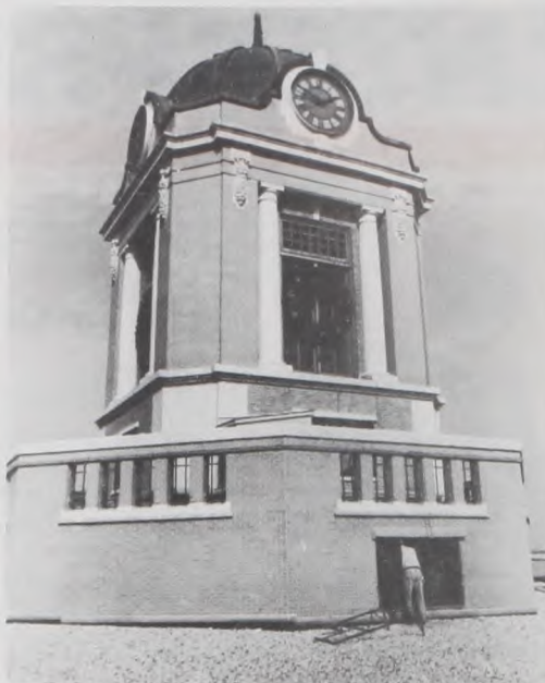
ATOP THE COOKE COUNTY COURTHOUSE - Capped by a copper covered dome, this brick covered drum graces the skyline of Gainesville as it has since the building's construction in 1911. Inside the windows are wreaths not yet down from the Christmas holidays. Each wreath is eight feet in diameter which might give some perspective on the size of this historic structure.
