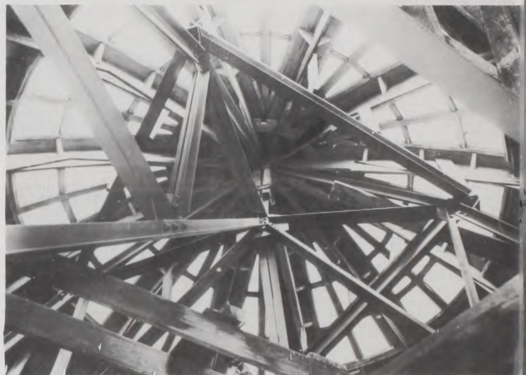
A RARE VIEW - the underside of the Cooke County courthouse's copper covered dome is the highest point inside the building. The intricate angles were necessary due to the dome's curves.
