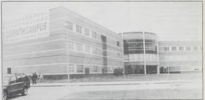
The new NCTC Corinth Campus main building is adjacent to Interstate 35 between Denton and Lake Dallas. Photo by Dave Fette
