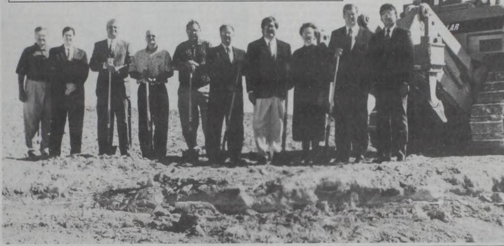
Officials from Ford Motor Company came to Muenster Friday morning to formally break ground for the new dealership home for Klement Ford of Muenster. Pictured left to right are Ray Nichols of Guaranty National Bank, David Mason and Gary Byrd of Ford Credit, Riley Peveto of Guaranty National Bank, Ron Bettis of J. M. Construction, Mike Daley of Ford Southwest Region, Karl, Edna, and Kirk Klement of Klement Ford, and Rick Barnes of Ford Muenster on Highway 82. Kirk Klement said the planned 32,000 square foot facility will open in July of 2000. Photo by Dave Fette
