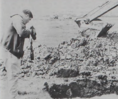
Doug Fleitman fills in a hole he just dug at the future Lake Muenster site. Above, Robert Gehrels, a physical science technician, video tapes the test pit for documentation. The holes are being dug to check soil material that will be used in building the dam.
