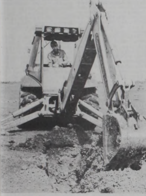
Doug Fleitman fills in a hole he just dug at the future Lake Muenster site. Above, Robert Gehrels, a physical science technician, video tapes the test pit for documentation. The holes are being dug to check soil material that will be used in building the dam.
